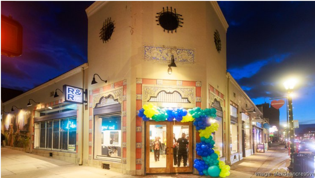
R&R Head Labs at 2260 East York Street
